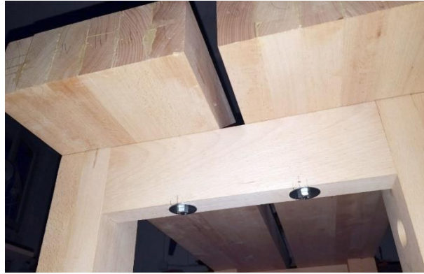
Lag bolts in place
